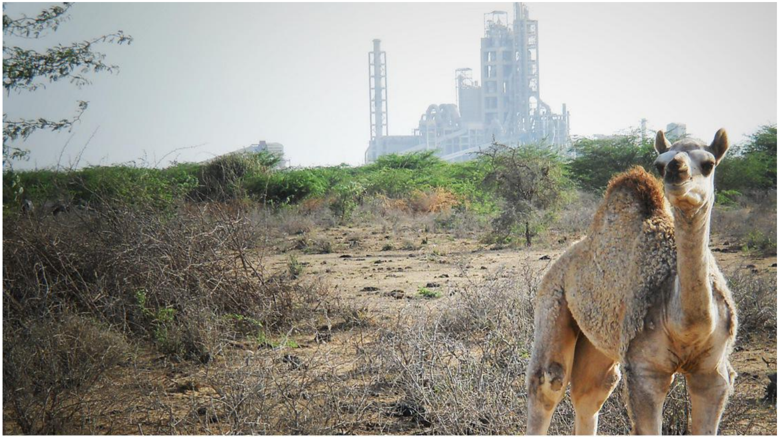
The Sanghi Cement plant is unmistakable against the skyline near Jadva village, Lakhpat taluka.
