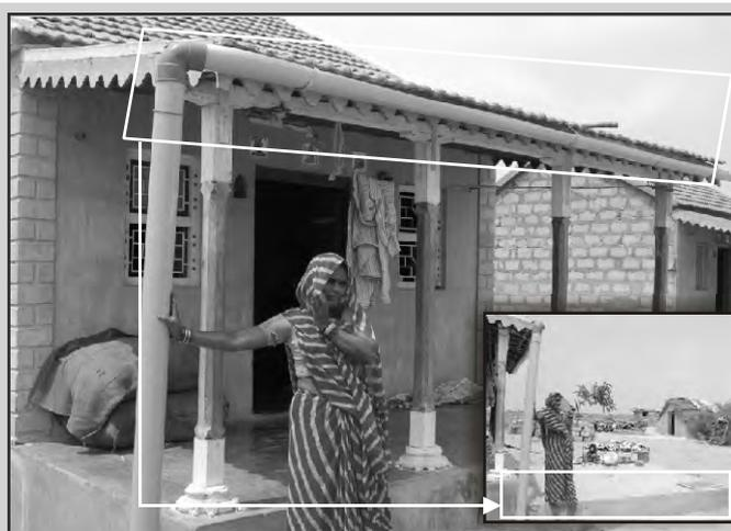
*In Pani Thiye Panjo programme, various technical and process innovations are being experimented. In Jethmalpar village every houses has rainwater harvesting tank which they use in stress condition. The concept of recharge bore well has been successfully demonstrated in some villages, pacca virda (very shallow dug well) has been constructed in Nimdivandh which is 500 meter away from the coast, whereas, solar pumping technologies are adopted by the villages*
