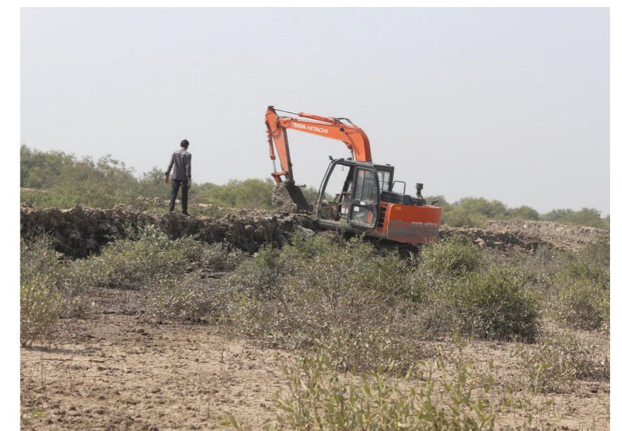
Trees from mangroves being uprooted. Picture credits: Hamir Jat
