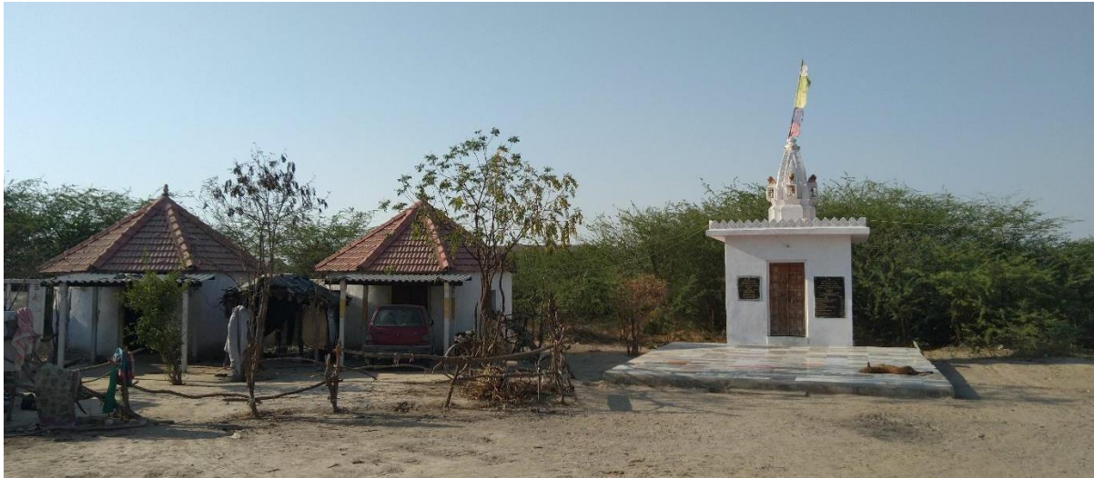
Fig 4: A typical Wadha settlement (permanent) with bhungas and a Ramdevpir temple. These were built through NGO support (RSS, Swami Narayan Trust and Vishwa Hindu Parishad).
